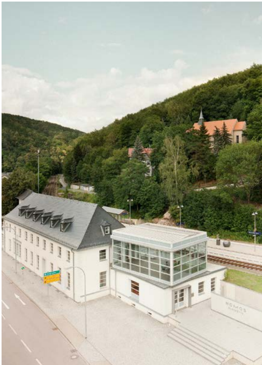
Nomos converted the old train station in the German watchmaking village of Glashütte into its HQ and factory, adding a glass-box boardroom with spectacular views of the surrounding Ore Mountains.
